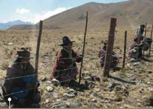
Community members install fencing
