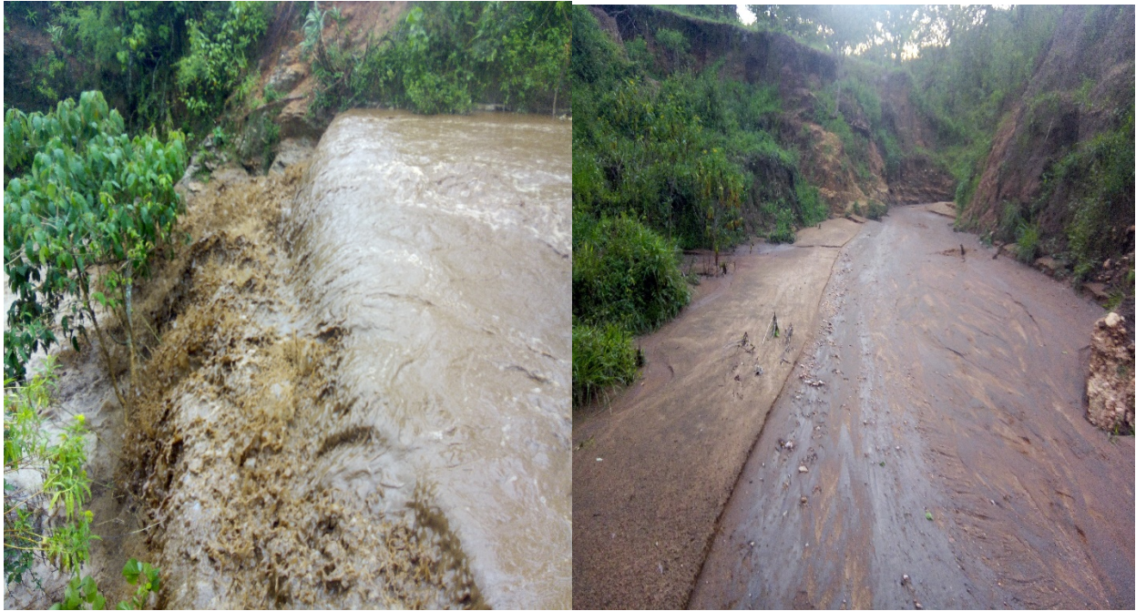
Figure 5. Sand dam providing physical barrier to water movement along the gully channel thereby (a) considerably reducing the speed of flash floods and (b) retaining sand.
