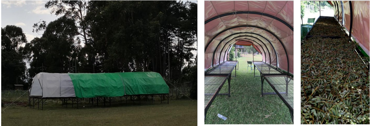
Figure 3: Locally fabricated structure to facilitate shade drying of pesticidal plants.
